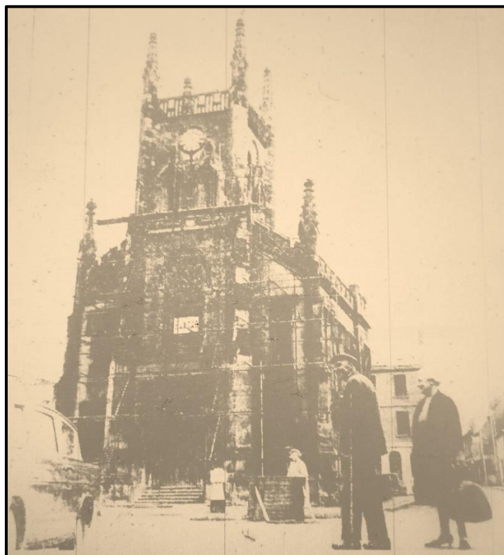
Scaffolding goes up around the town hall, ready for demolition, June 1966
