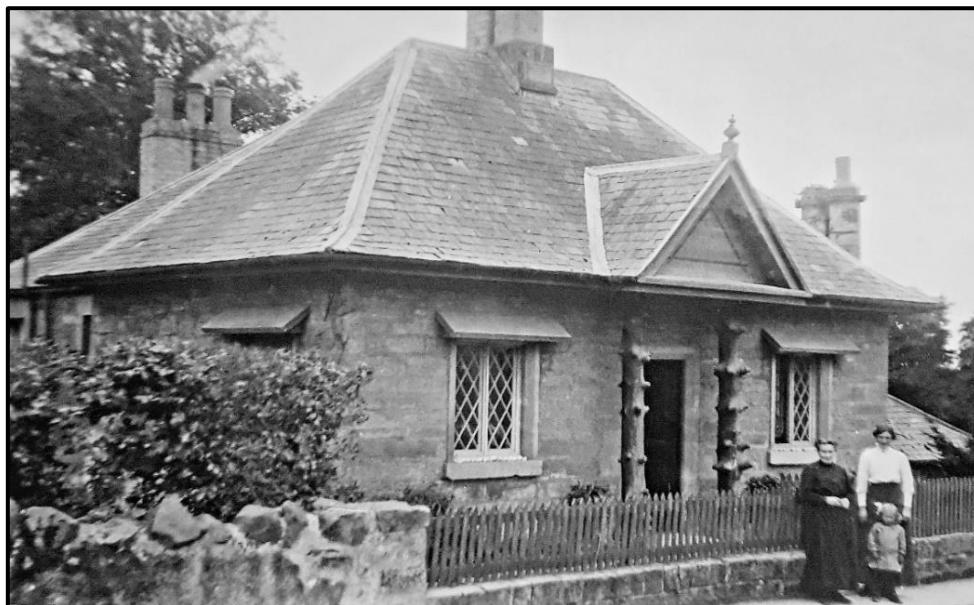
Wellfield Cottage before the Great War; the porch was later removed and the doorway blocked up, probably since the house frontage was so close to the road
