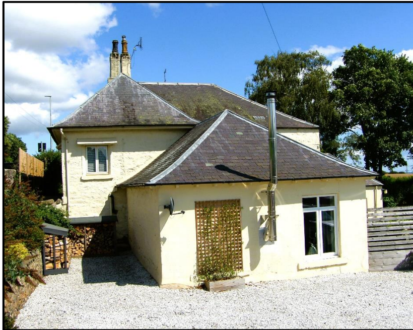
West elevation of Far Ben (originally Wellfield Cottage)
