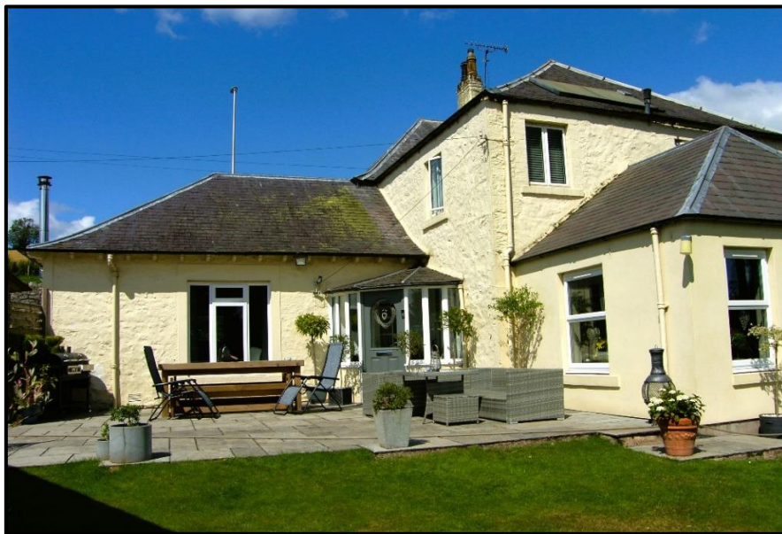
Apart from the sun room (far right), the house footprint is largely original
