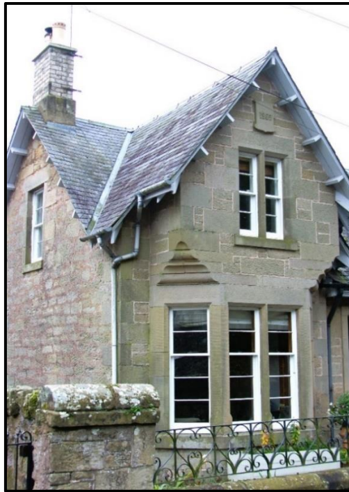
North elevation with corbelling and 1865 date stone
